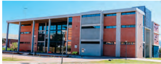
Pictured: The new building at DUT's Indumiso campus.
